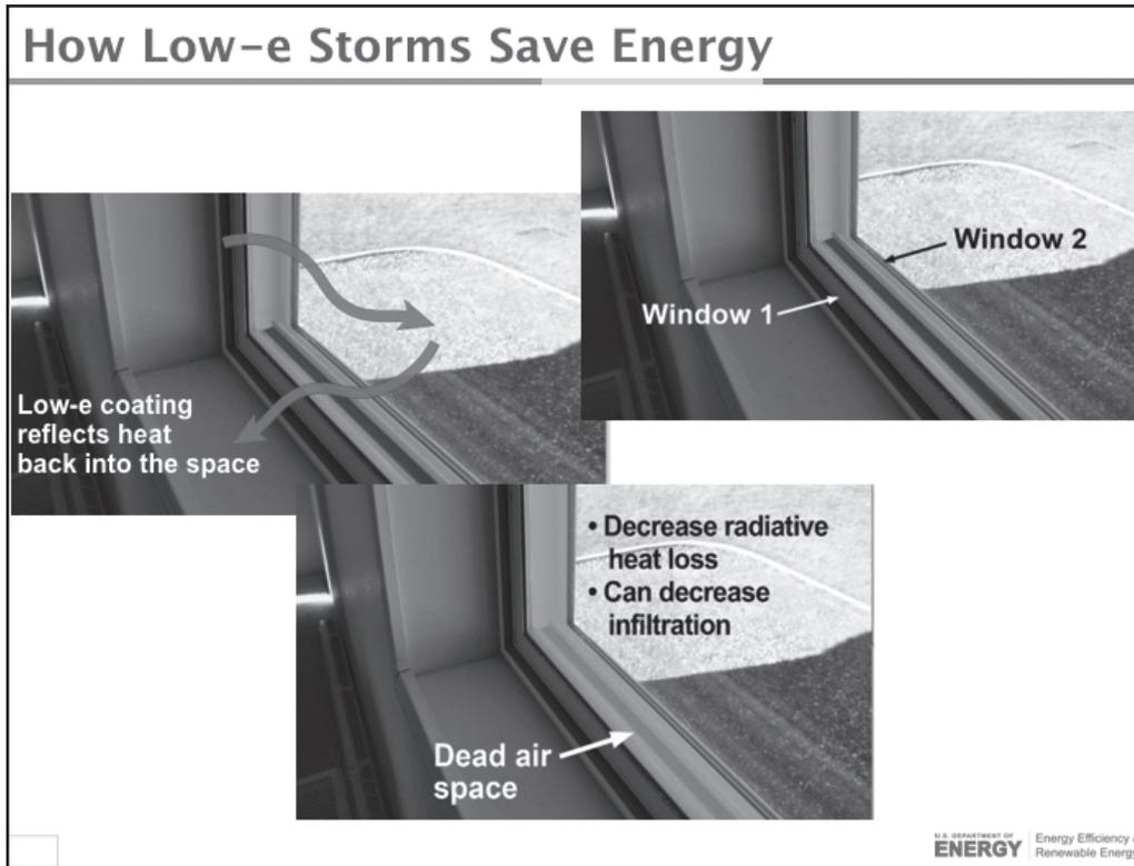
Figure 2. How Low-E storm windows save energy. Figure courtesy Sarah Widder, the Pacific Northwest National Laboratory, and the US Department of Energy, Energy Efficiency & Renewable Energy.
