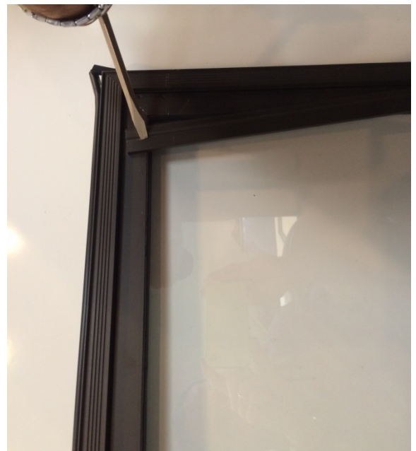
Figure 2: Remove Header Locking Bar
